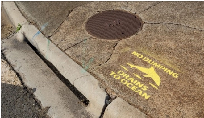
Figure 2: Stenciled Storm Drain at MCBH
